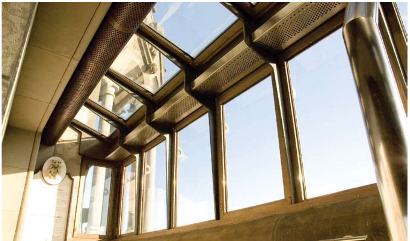
Looking up through the weather resistant projected window enclosure system
