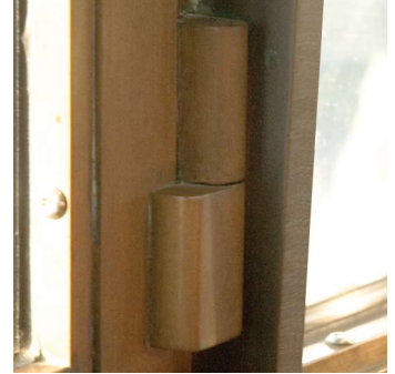
Alloy 230 custom made red brass hinges
