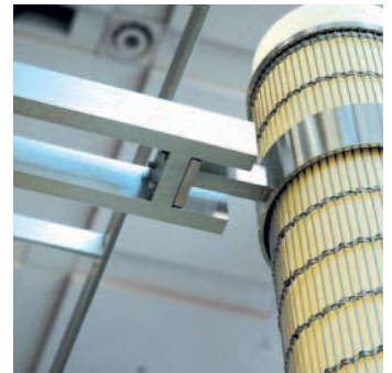
Light fixture connection details
