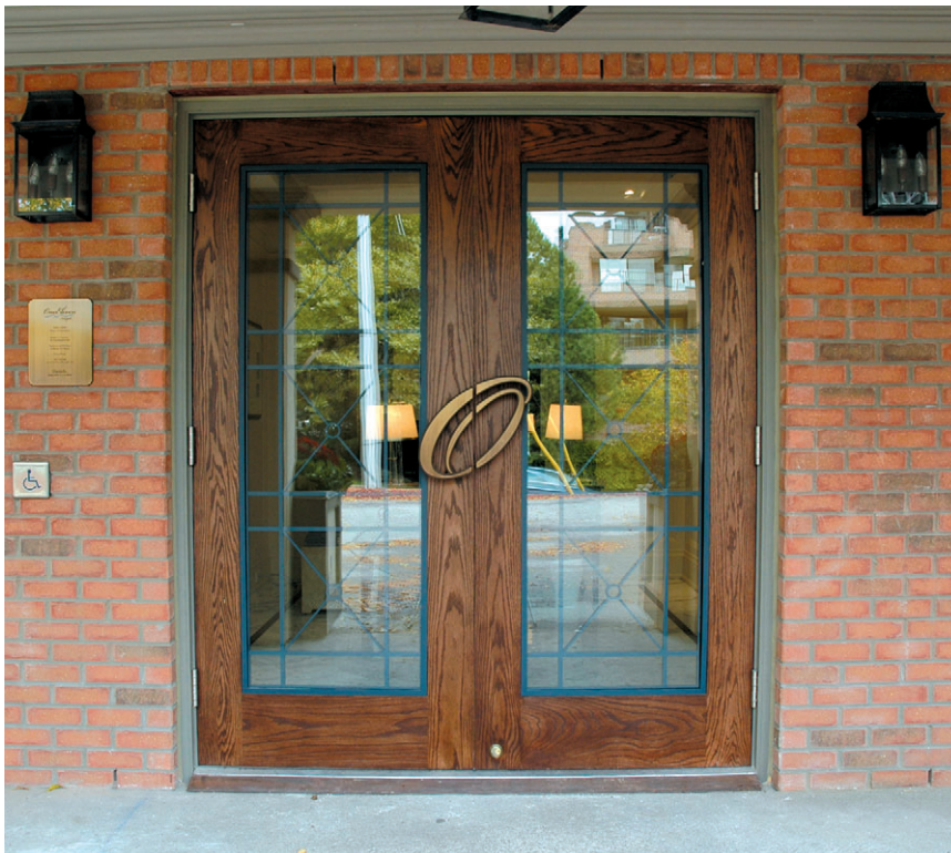
Main front door glass and grill inserts
