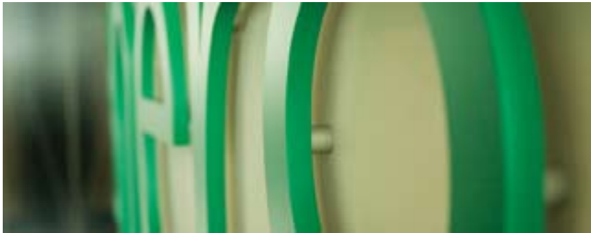
Detail of the pinned mounting system on the precision cut acrylic text graphics
