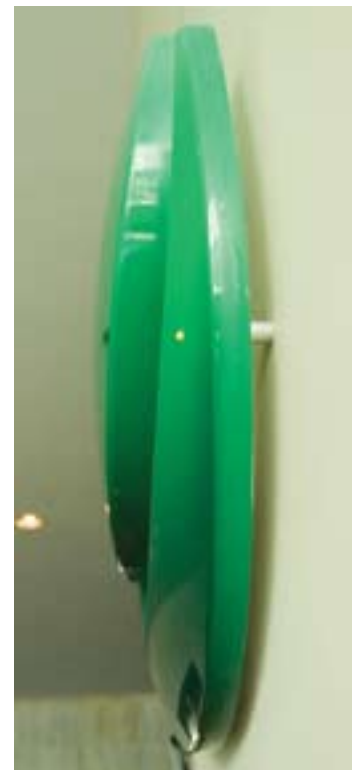
Pinned mounting viewed from beneath
