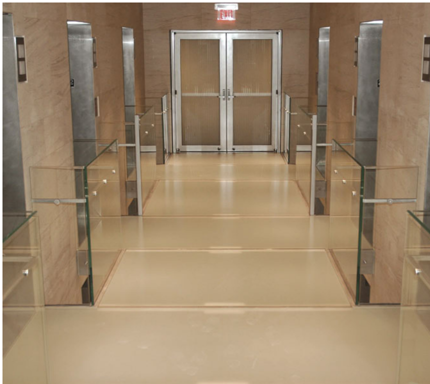
Glass bridge services elevator entrances
