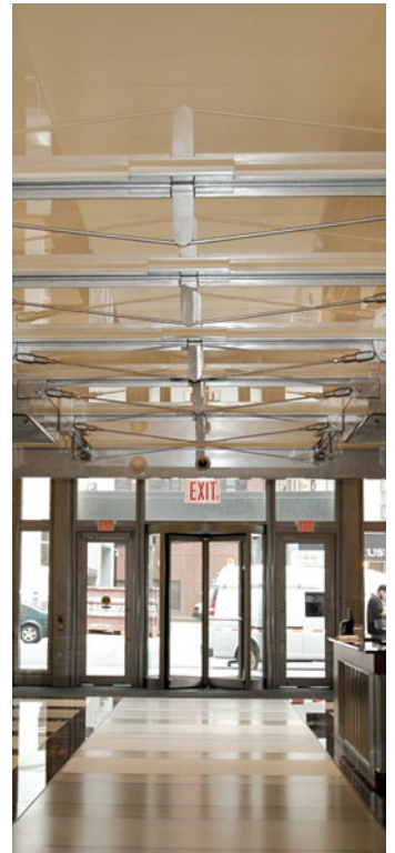
Underside of bridge view
