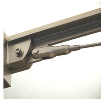
Clevis jaw hardware detail
