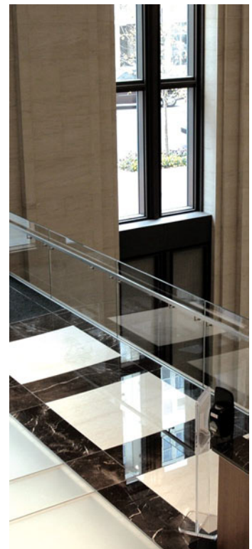
Glass floor and balustrade from above
