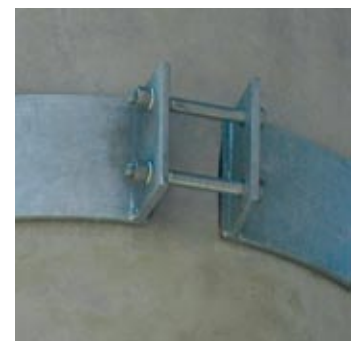
Solid, bolted lap joint connection
