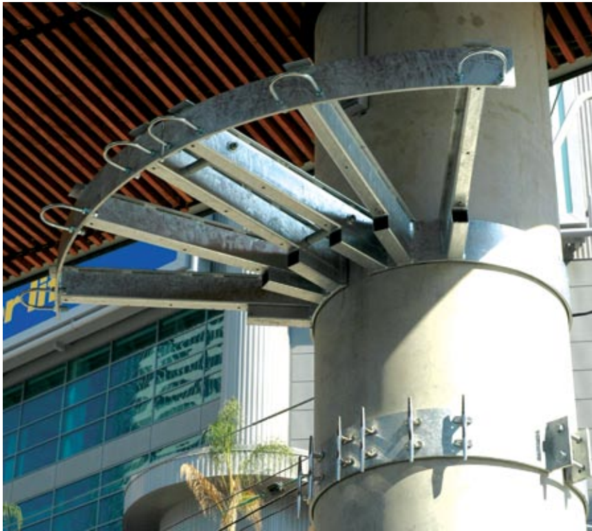
Custom steel column brackets used for the specialized suspended lighting system at the 2008 Luminato® Festival in Toronto
